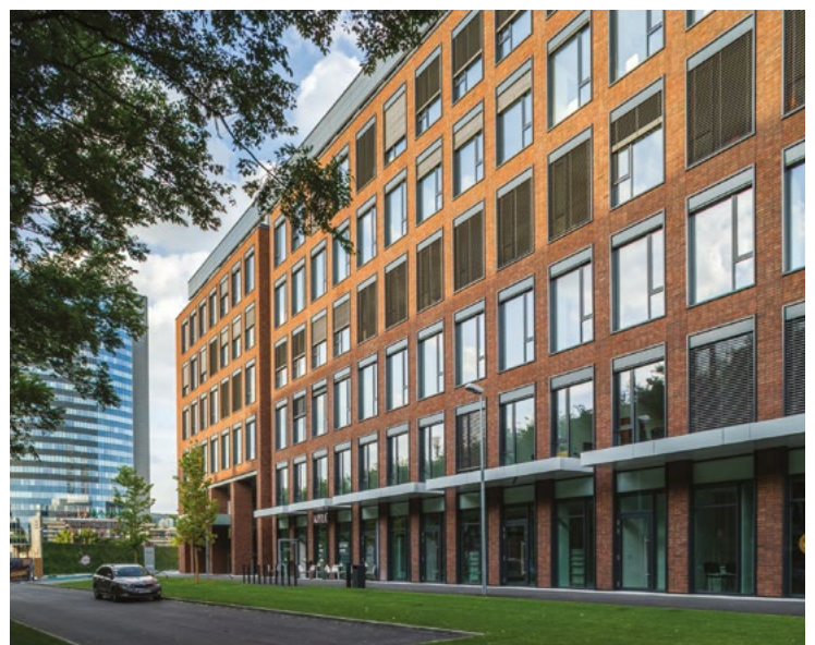
Completed Twin City
